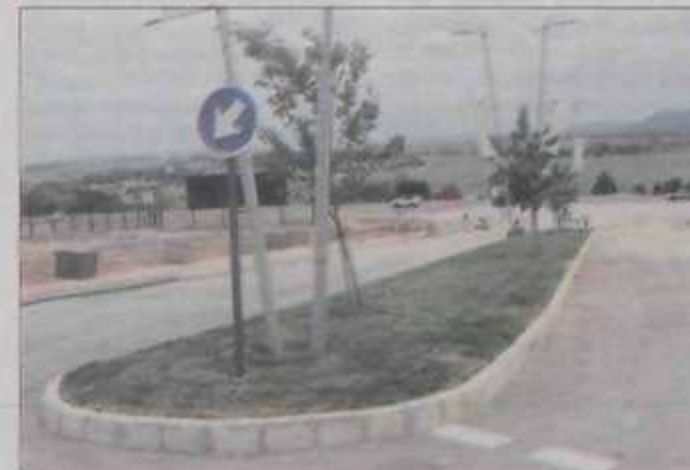
SMOOTH: Road upgrades near Lanseria Corporate Estate.
